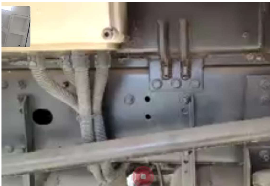
Picture-3 Bolting of chassis of vehicle and beam of Sky lift
