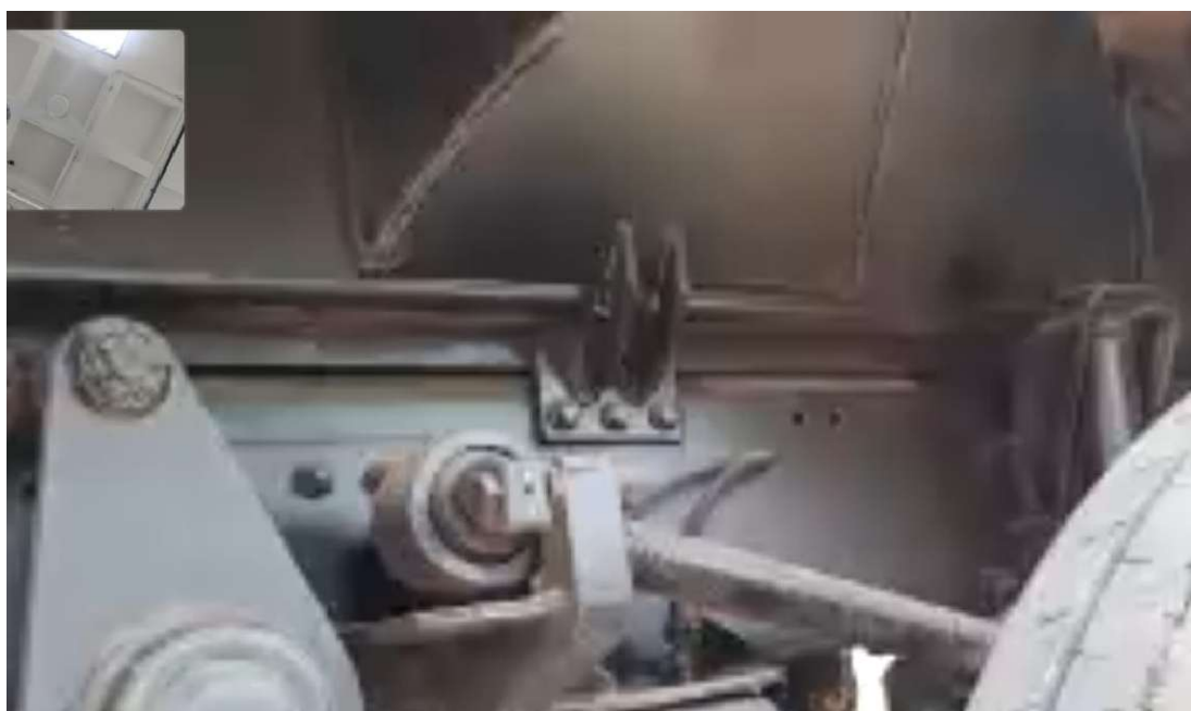
Picture-4 The bolting of the Skylift with the back side of the chassis
